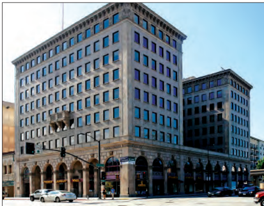
Purchased: Beaux-arts property at 234 E. Colorado Blvd.
