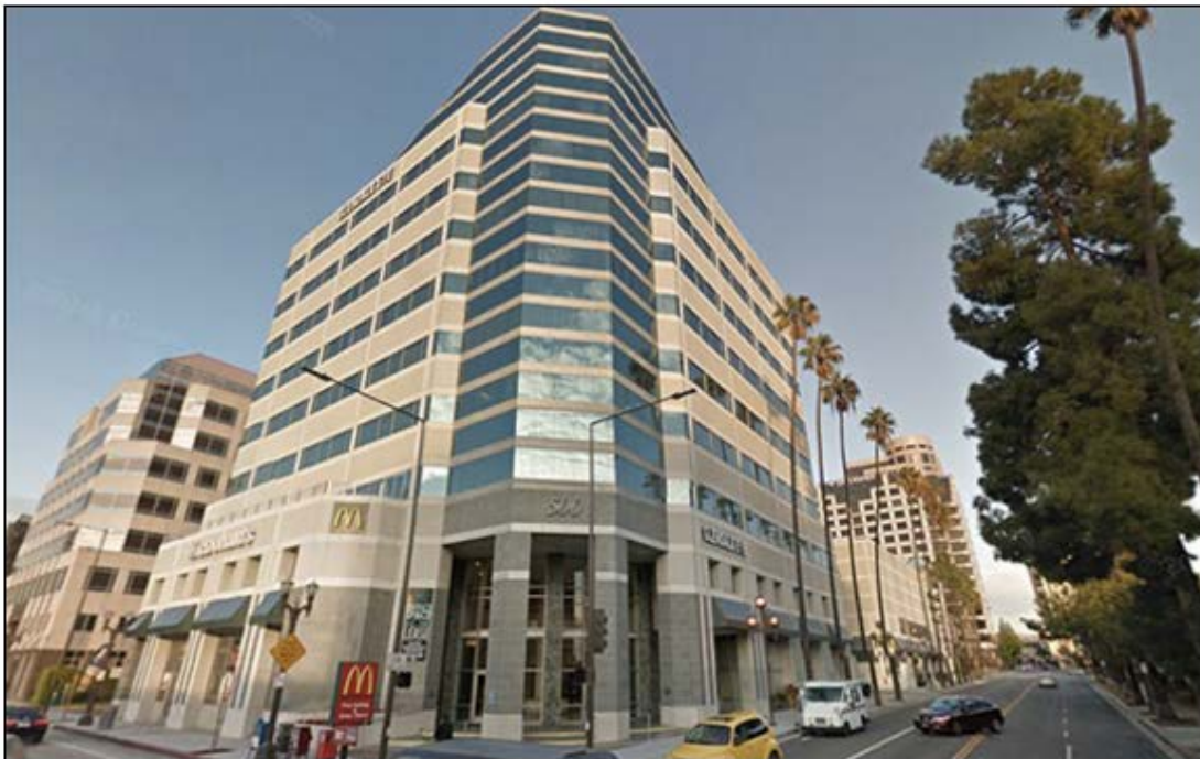
The office building at 500 North Central Avenue (credit: Google Earth)
